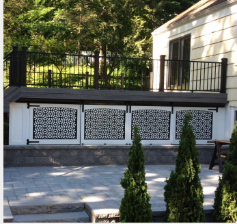
Custom Skirting Around Deck Perimeter
